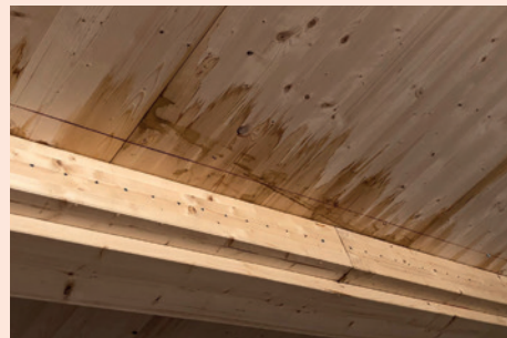
Building damage through wetness
